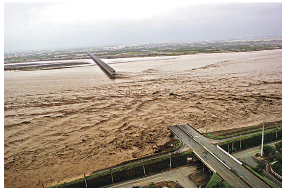
Fig. 1 Collapse of Shuangyuan Bridge (2009/8/10) (photo courtesy of Apple Daily)
