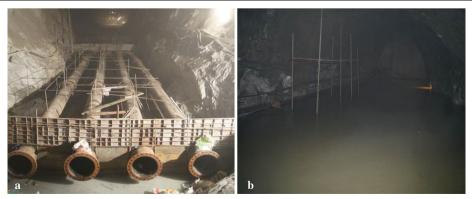
**Fig. 9** Drainage measures in the diversion tunnel: **a** installing of drainage pipe and **b** water catchment in the drainage tunnel before draining
