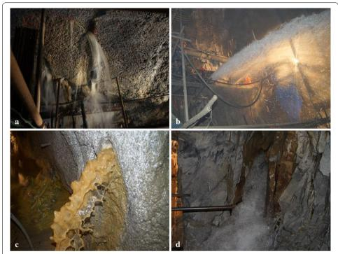
**Fig. 5** Water inrush disasters in the diversion tunnel during the construction process: **a** low flow water inrush; **b** large flow water inrush; **c** water inrush with silt; and **d** water inrush from a structural surface
