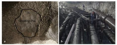
**Fig. 12** Groundwater plugging measures at water inrush points: **a** grouting technology for plugging; **b** caisson technology for groundwater treatment
