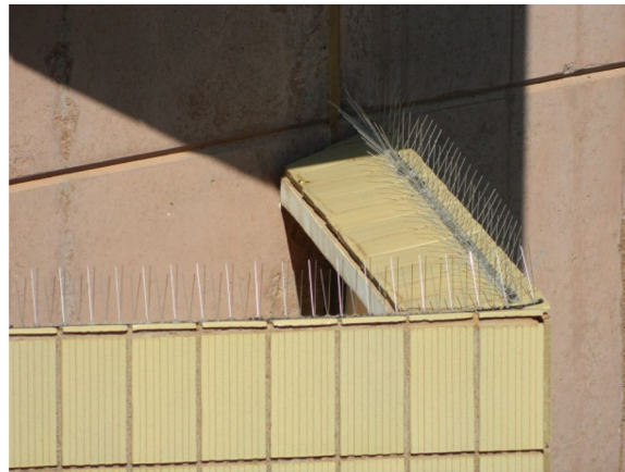
Fig. 4 Bird spikes evaluated as a pigeon deterrent on the University of South Africa's Muckleneuk campus
